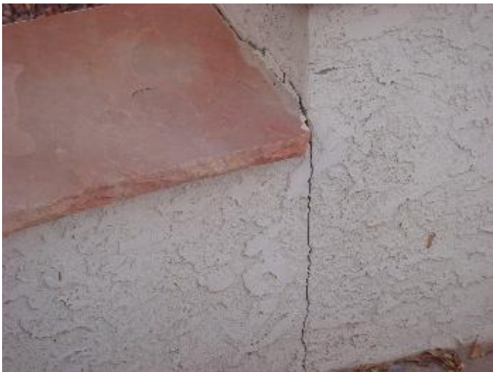
Vertical crack through stucco on rear seating area
